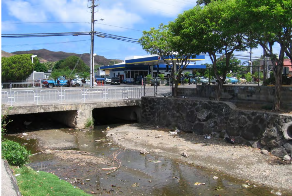
Photo 1-28 Hele Drainage Channel and twin Keolu Drive box culverts. Note RCP coming in from Enchanted Lakes Shopping Center to the right (south).
