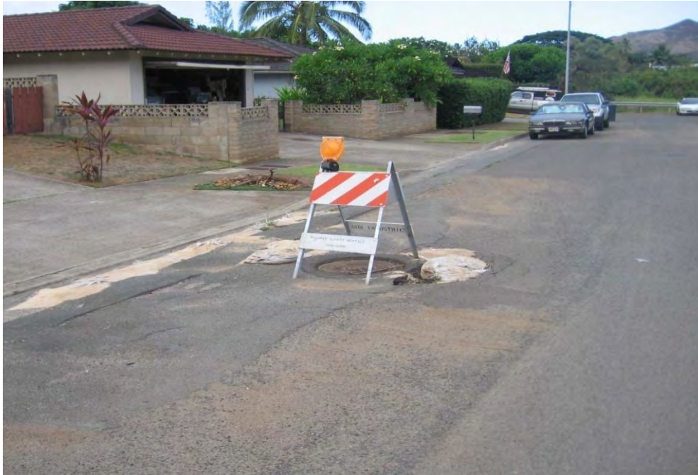
Photo 1-53 Storm drain manhole on Akumu Street is frequently popped during storm events due to back pressure from WKIP 43 outlet blockage and 90-degree alignment bend at this junction.
