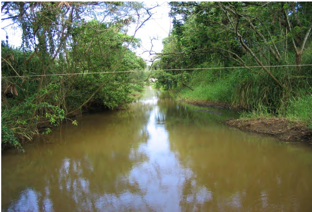
Photo 1-40 Unlined portion of Keolu Drainage Channel.
