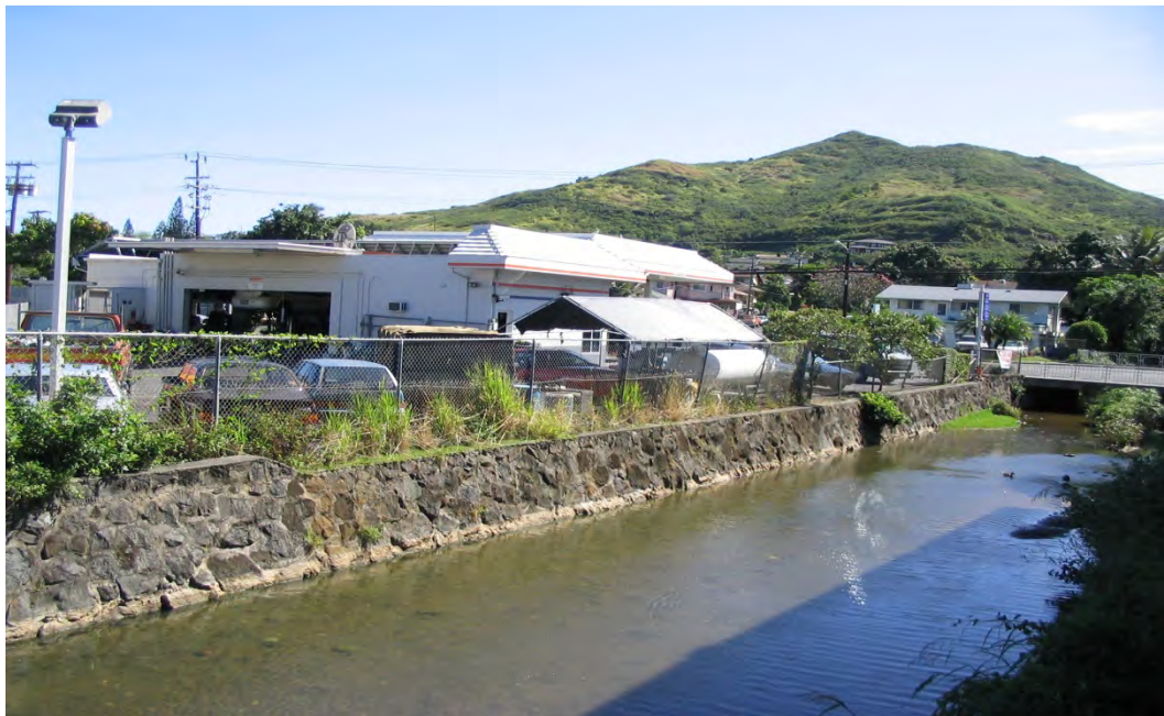
Photo 1-27 Hele Drainage Channel looking upstream toward Keolu Drive. Note: previous location of Tenn's Service Station
