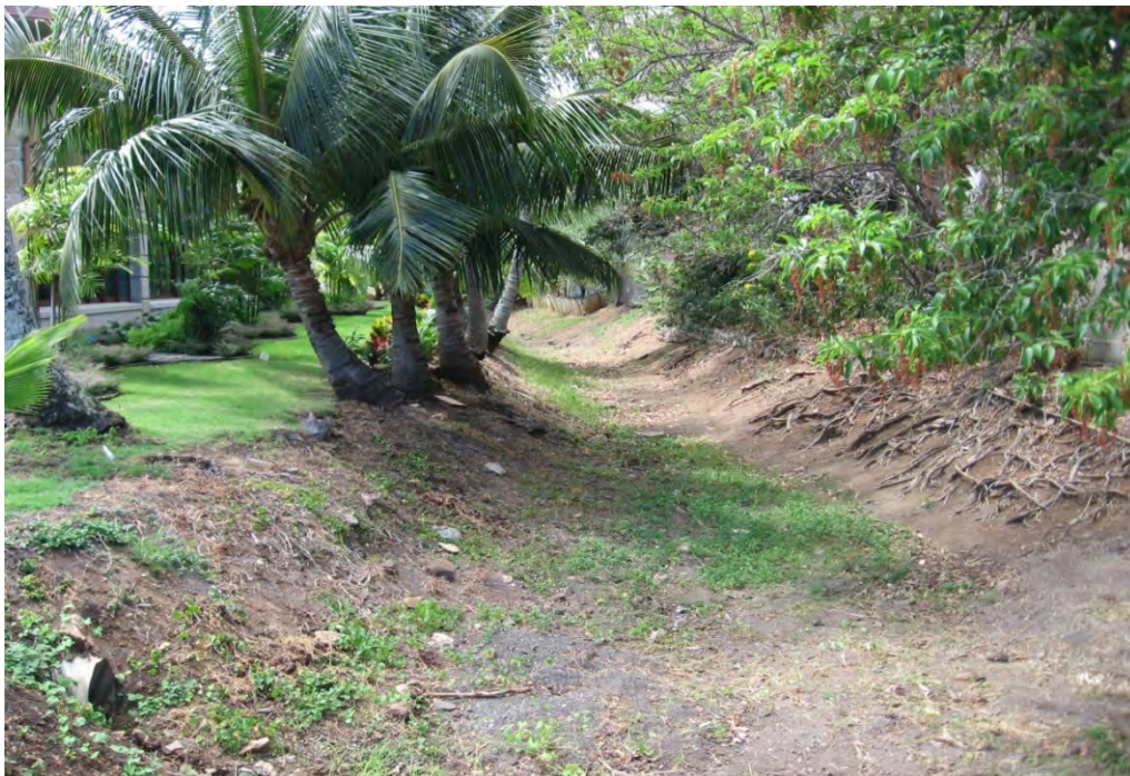
Photo 1-22 Kamahele earthen ditch looking southwest from Keolu Drive. Note scouring of embankment, road debris accumulation in the ditch, and church drainpipe outlet .
