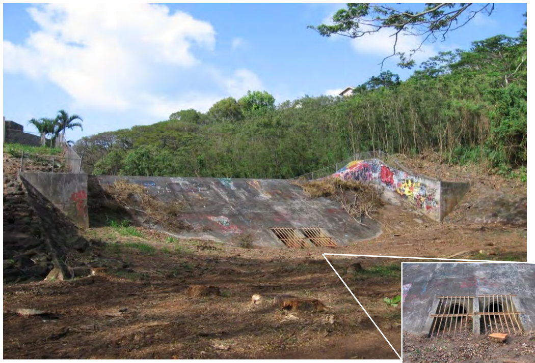
Photo 1-46 City debris control system at beginning of Keolu Lined Channel. Note recently cleared area with debris scattered. Grated inlet houses two 18-inch RCPs.
