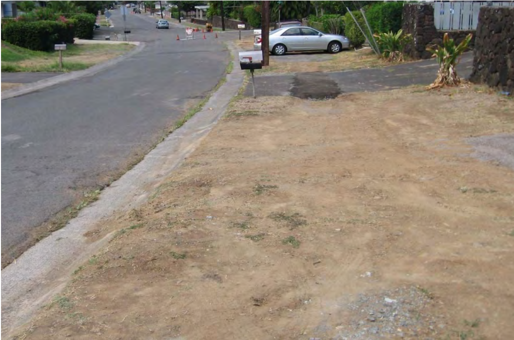
Photo 1-35 Road construction and barren area on Hele Street looking northwest. A typical scene within this drainage area and others in the study.
