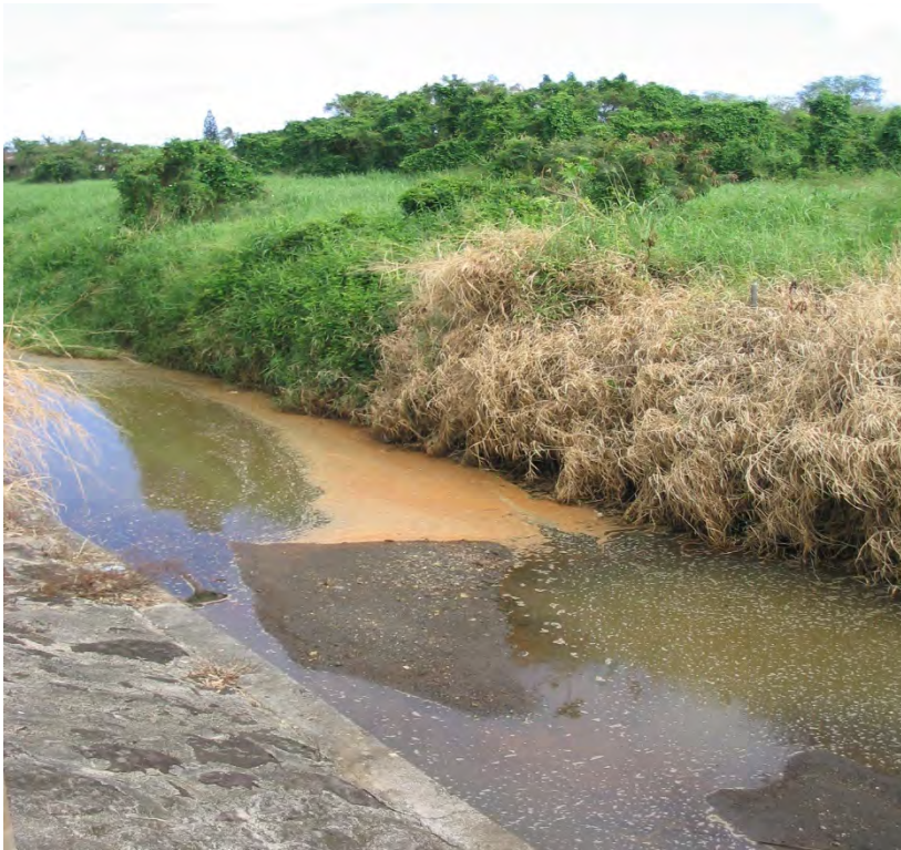
Photo 1-41 End of Keolu Lined Channel and beginning of unlined portion of channel. Note this area is typically stagnant, even during significant flows (see following photo) due to increased depth from scouring of unlined channel bottom.
