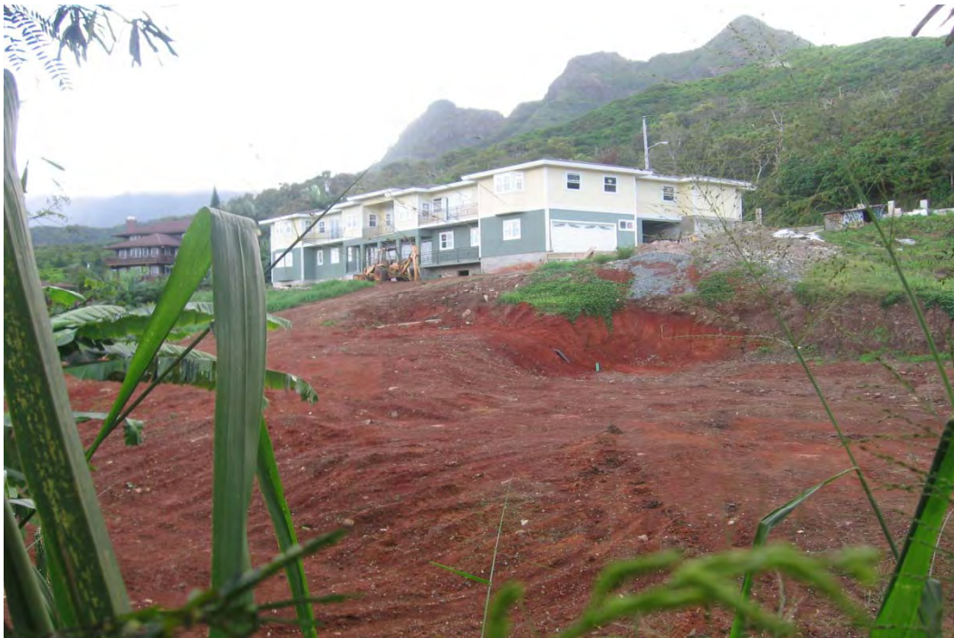
Photo 2-1 Construction site along Old K-Hwy. Structural BMPs were not observed on site. Photo taken from K-Hwy.
