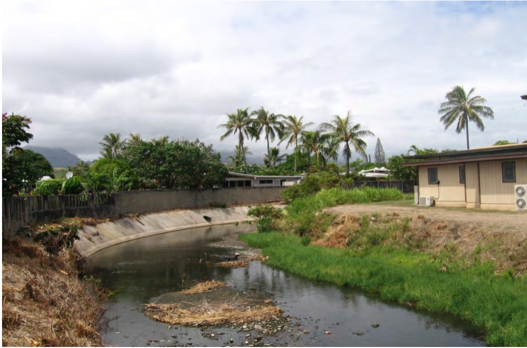
Photo 1-26 Hele Drainage Channel looking downstream. Note large Mango Tree, Alahaki Street outlet, sediment deposits with vegetation growing on the north bank, gross debris within channel, and dead grass (sprayed) on south bank.
