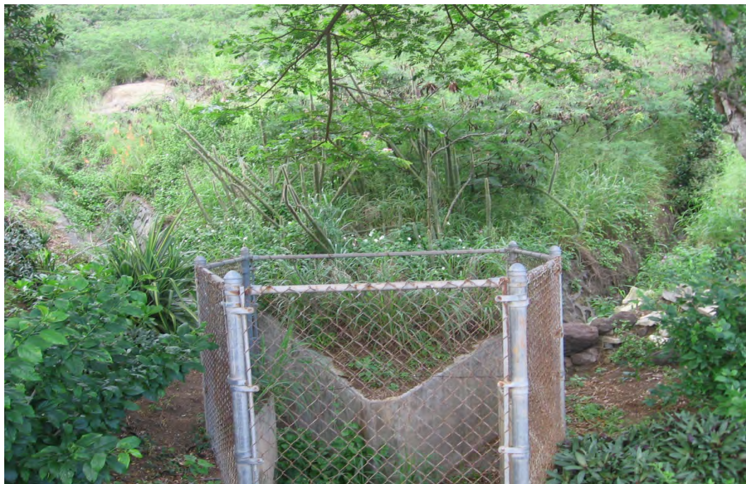
Photo 1-14 showing lined drainage ditch collection system from the hill behind Akiohala Place.
