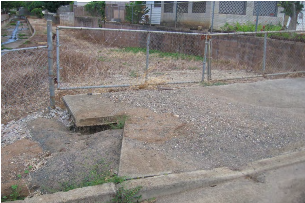
Photo 1-54 Erosion and sediment deposits at the end of Akumu Street. Note Keolu Lined Channel and City access easement in background.
