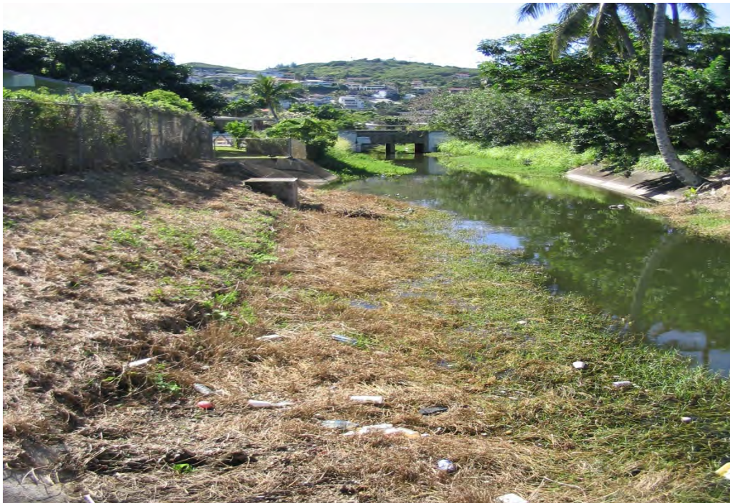
Photo 1-2 Alahaki Ditch looking upstream toward Kahili Street Bridge. Note Interceptor Ditch #1 junction and excessive dead vegetation from spraying.
