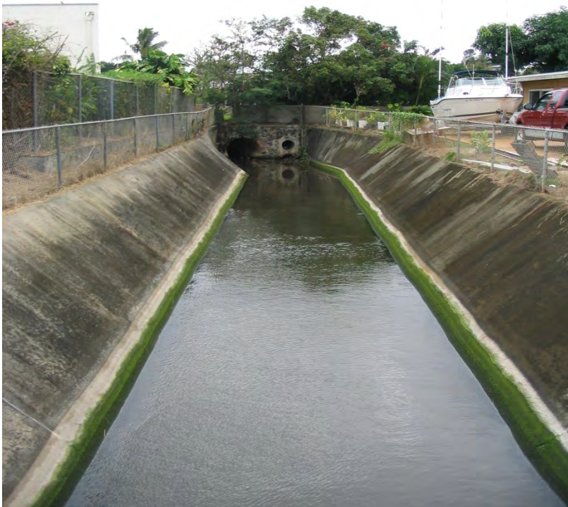
Photo 1-4 Photo taken from Alahaki Street Bridge looking northeast (upstream) of Interceptor Ditch #1. Note corner of movie theater from Enchanted Lake Shopping Center, relief drain and pipe from Keolu Drive.
