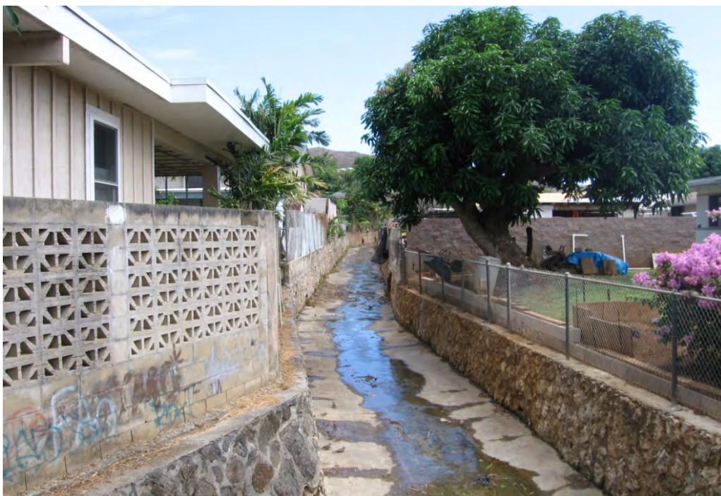
Photo 1-31 Hele Drainage Channel looking east from 6 th parcel from Liku Street Bridge. Two RCPs (24 and 36-inch) come in from Loho Street here.
