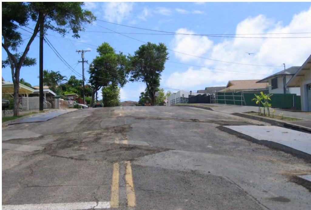
Photo 1-34 Road construction on Loho Street looking southeast.
