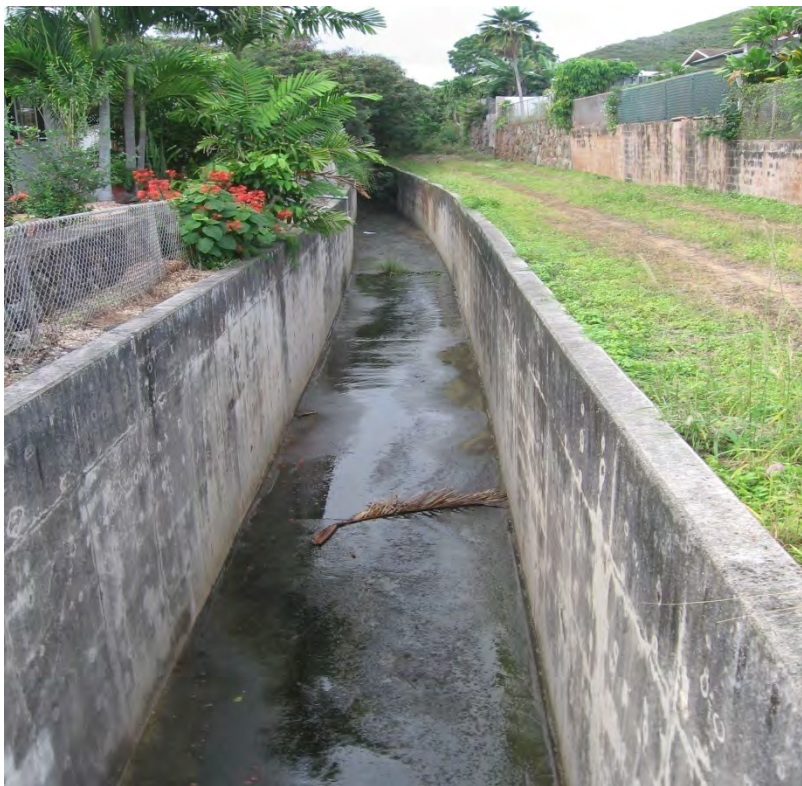
Photo 1-10 Akipola Lined Channel looking upstream. Note: City and County maintenance easement extends to beginning of channel.
