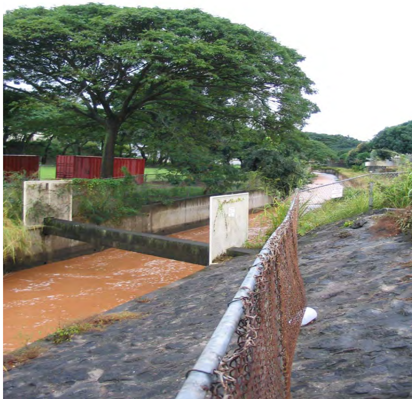
Photo 1-42 Keolu Lined Channel after an April 2005 storm event looking upstream (southeast) with Keolu Elementary School on its eastern border.
