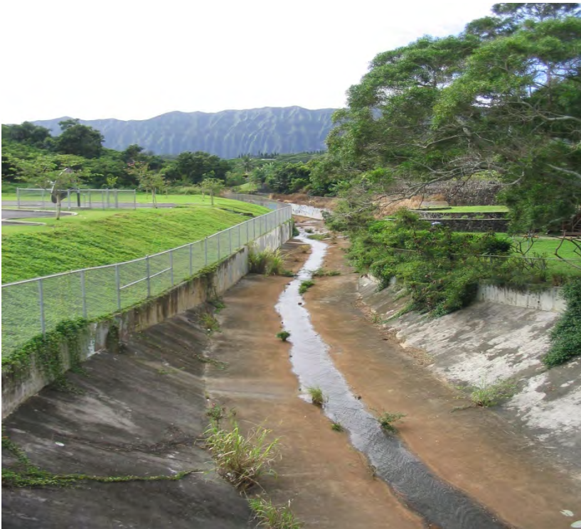
Photo 1-44 Keolu Lined Channel looking upstream (south) from Keolu Drive.
