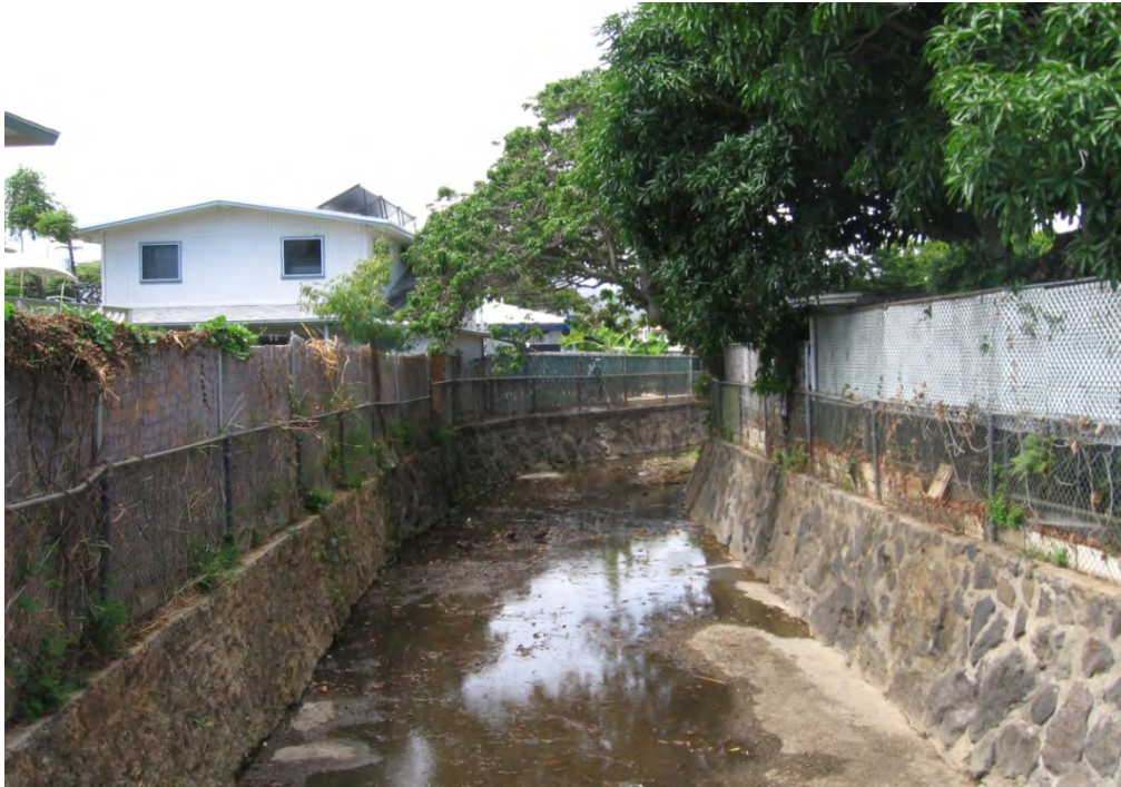
Photo 1-30 Hele Channel looking east from Liku Street.
