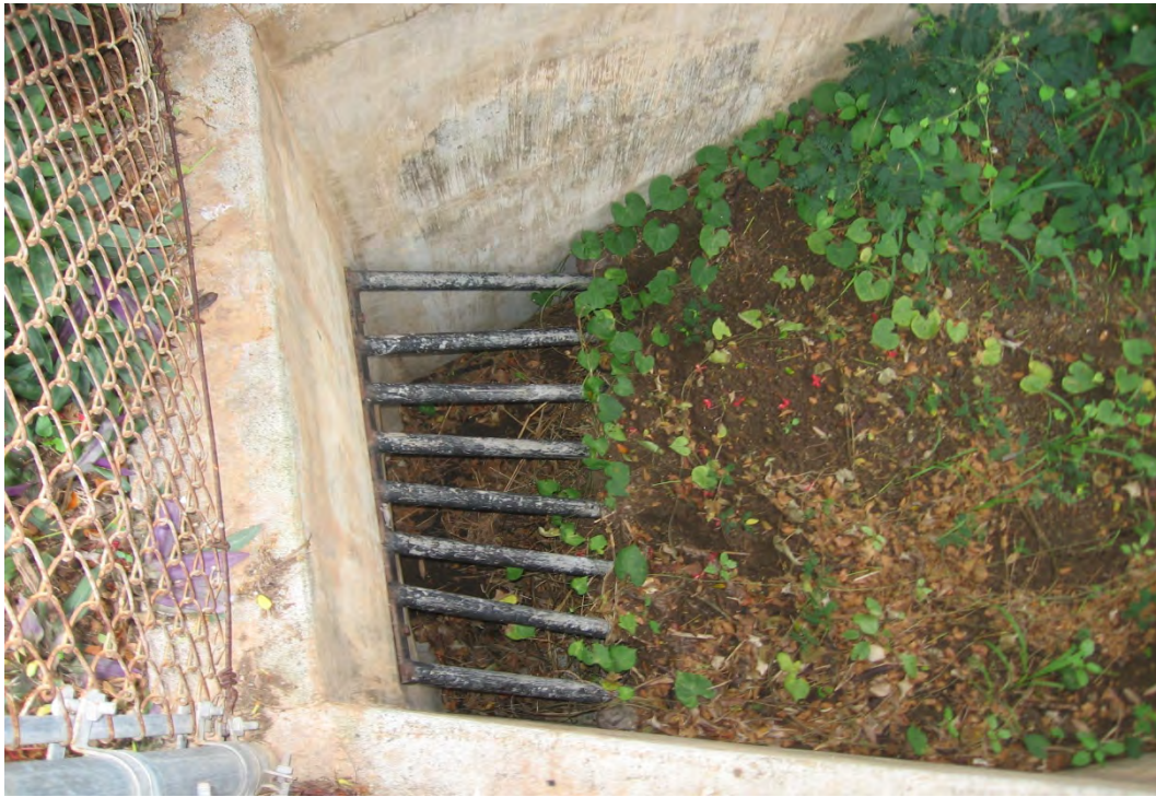
Photo 1-15 vegetation screening bars at intake pipe from lined ditch collection system at Akiohala Place.
