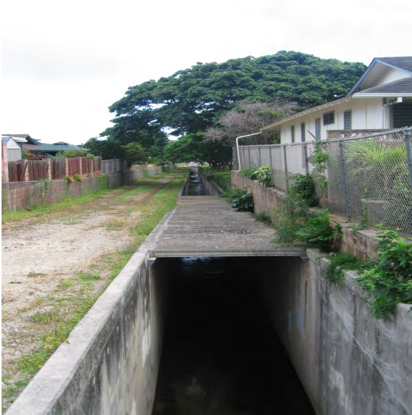
Photo 1-9 Akipola Lined Channel looking downstream. Note: concrete covering over this section of the channel helps reduce green waste buildup in the channel.
