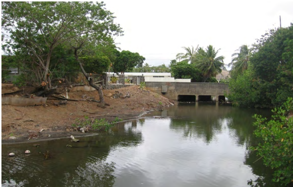
Photo 1-18 WKIP 10, Hele Channel looking north at Akumu Street Bridge from Kamahele Ditch junction. Note sediment build up and barren embankment. Recommended bank stabilization area using vegetative riprap and/or mechanical revetment .
