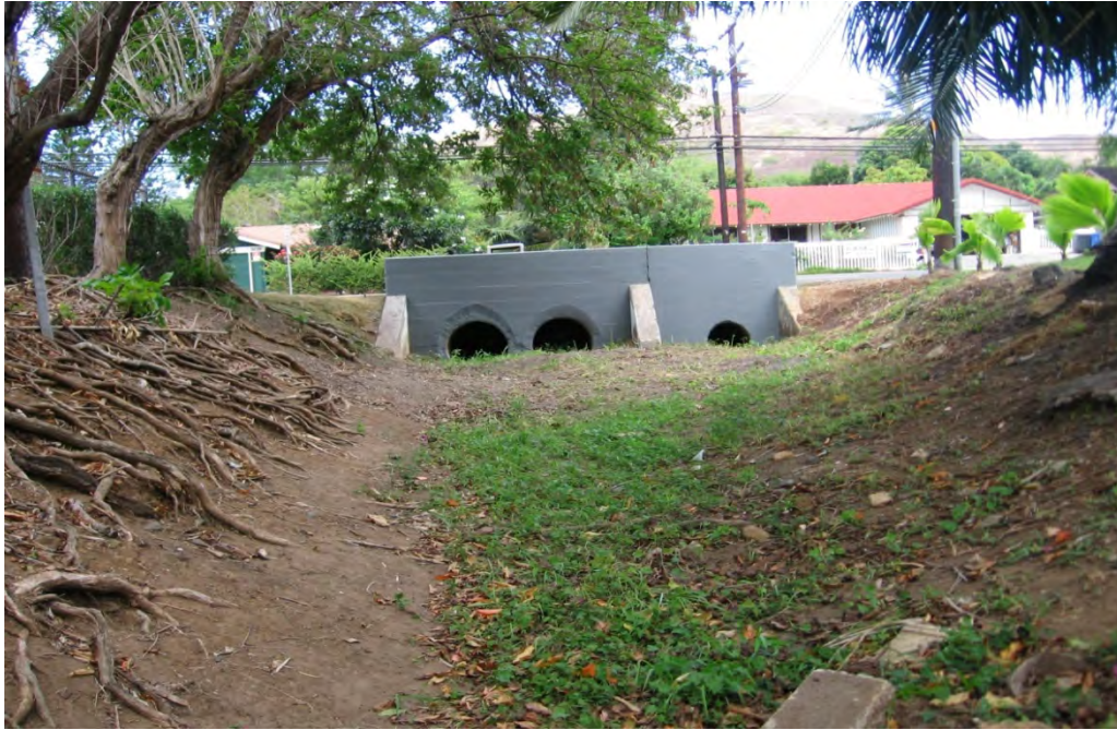
Photo 1-21 Kamahele Ditch looking northeast toward Keolu Drive. Recommended area for ditch excavation of deposited soils and bank stabilization (both sides) using vegetative riprap and/or mechanical revetment.
