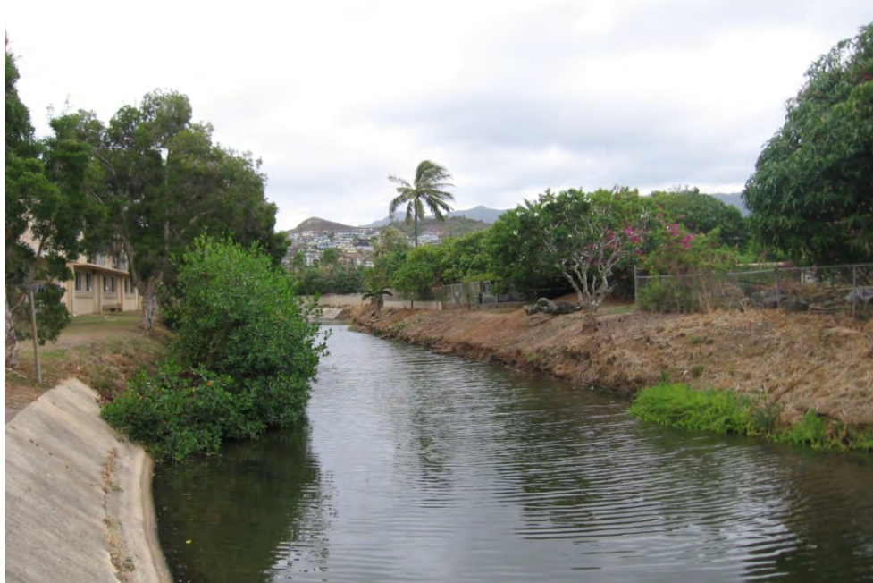
Photo 1-25 WKIP 10 Hele Drainage Channel looking south from Kamahale Ditch junction. Note erosion of unlined channel bank. Recommended bank stabilization area using vegetative riprap and/or mechanical revetment.
