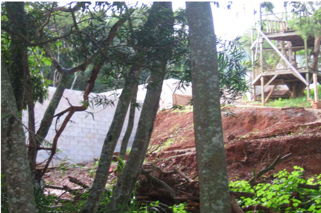
Photo 2-2 Construction site along Old K-Hwy. Structural BMPs were not observed on site.
