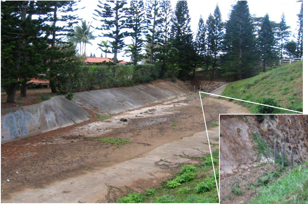
Photo 1-55 Concrete lined silt off of Old Kalaniana'ole Highway, which is part of WKIP 34 outlet discharging into Kapaa Silt Basin.
