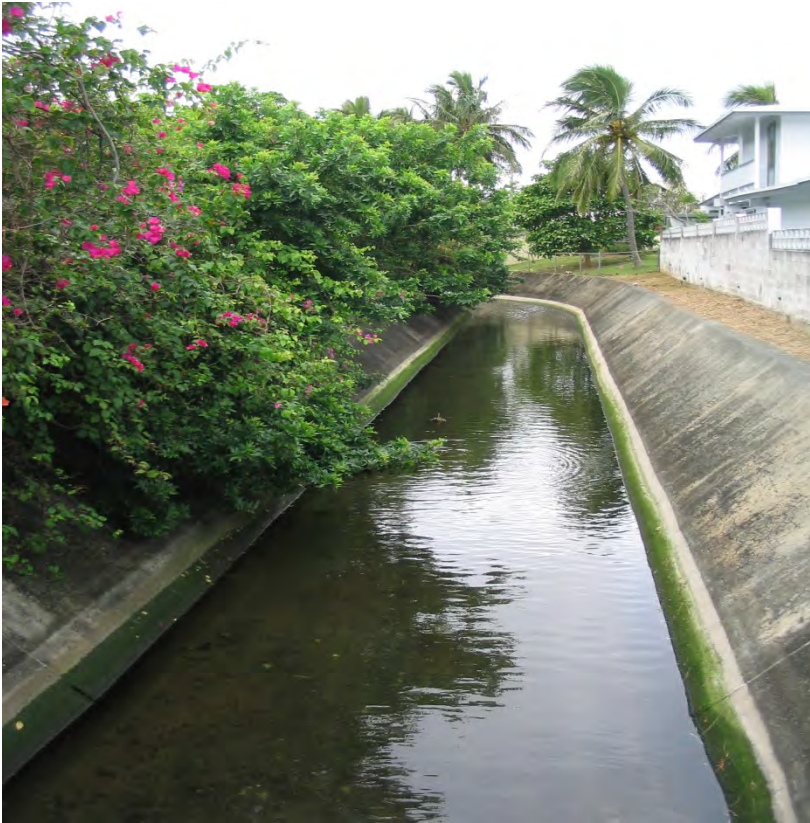
Photo 1-3 Photo taken from Alahaki Street Bridge looking northwest (downstream) of Interceptor Ditch #1.
