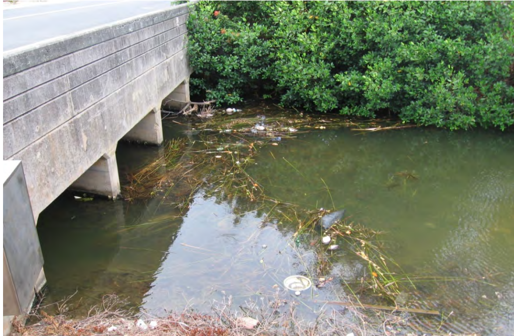
Photo 1-37 WKIP 10 drainage area Akumu Street Bridge. Potential location for vegetation screening bars.
