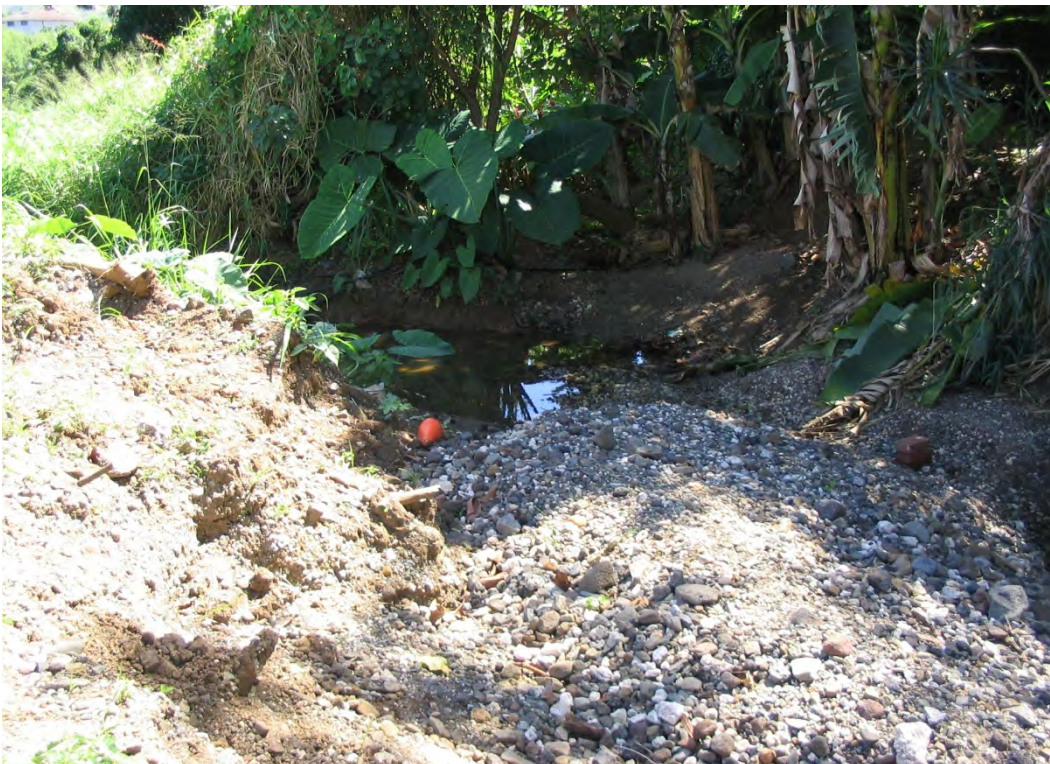
Photo 1-52 WKIP 43 outlet buried by sediment and debris.
