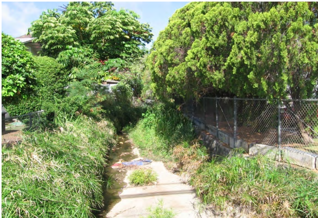
Photo 1-29 Hele Drainage Channel looking east from Keolu Drive. Tenn's Auto is the property adjacent to the south.
