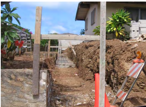
Photo 1-57 Residential construction site on Keolu Drive without BMPs. Pollutant source area for storm water runoff into WKIP 42 drainage system.
