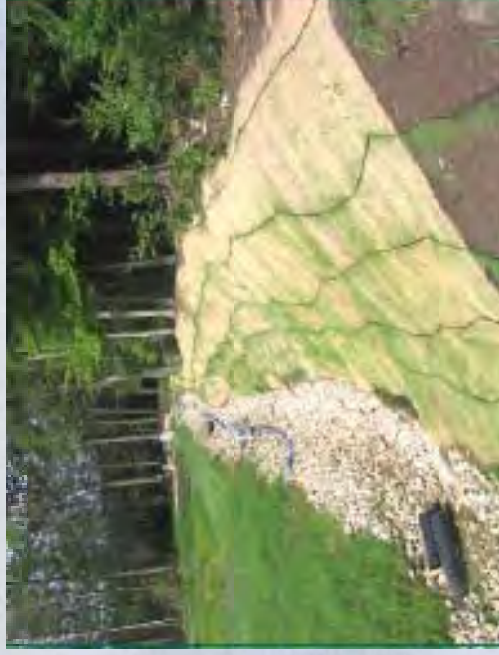
Vegetative swale, can be implemented to retain sediment and decrease velocity of stormwater runoff.
