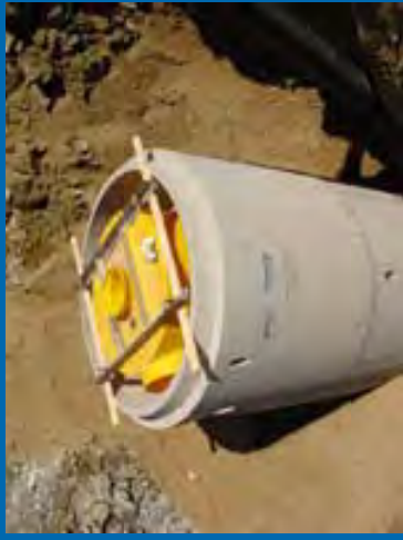
The Downstream Defender submerged inlet w/out weir or orifices enclosed in a Concrete storm drain (insert).
