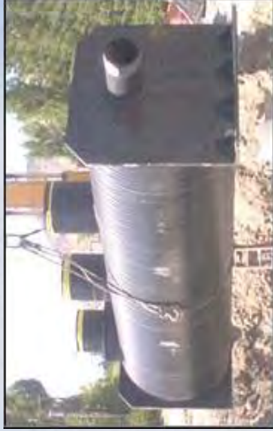
The Aqua-Swirl and Aqua-Filter, using the process of vortex and filtration to remove contaminants from storm water.
