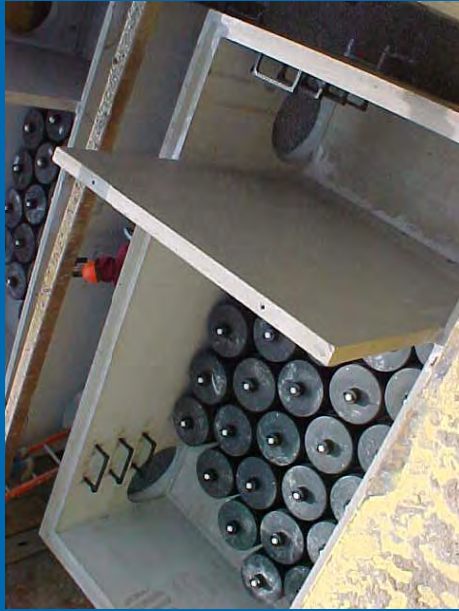
The StormFilter manhole/vault configuration.
