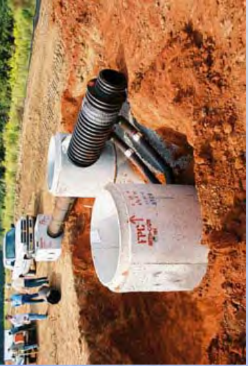
The BaySaver® implements two (2) manholes for controlling storm water quality.
