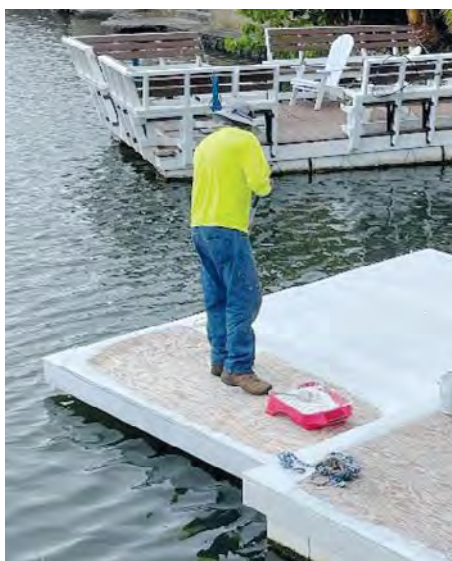
Sean added waterproof coatings to the barges.
